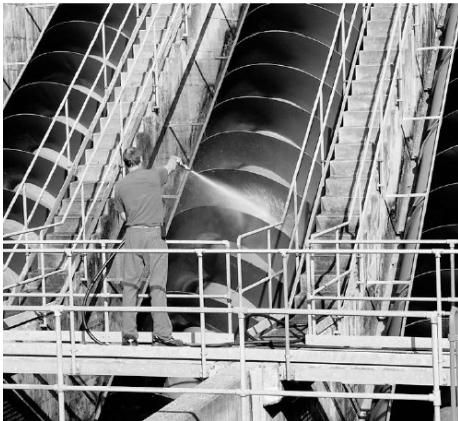
Energie in ARA
